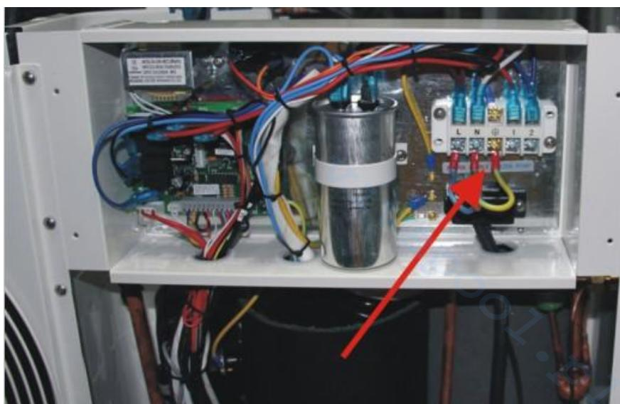
Note: In the case of three-phase models, swapping two phases may cause the electric motors to run in the reverse direction, which can lead to damage. For this reason, the unit has a built-in protective device that breaks the circuit if the connection is not correct. If the red LED above this safety device lights up, **you must swap the connections of two of the phase wires.**
